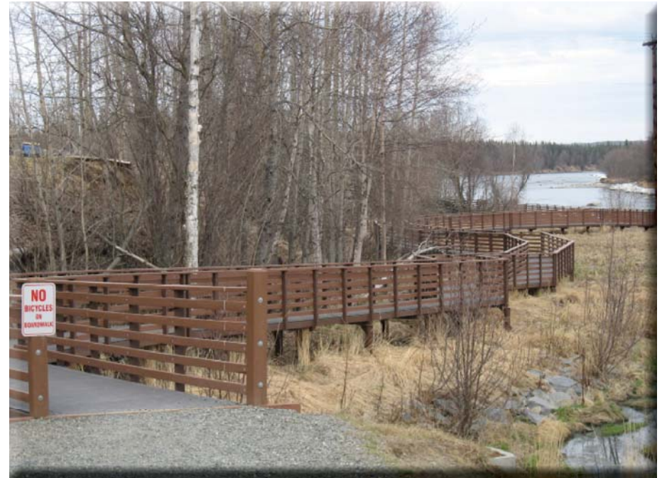
Kenai River boardwalk behind the Aspen Hotel
