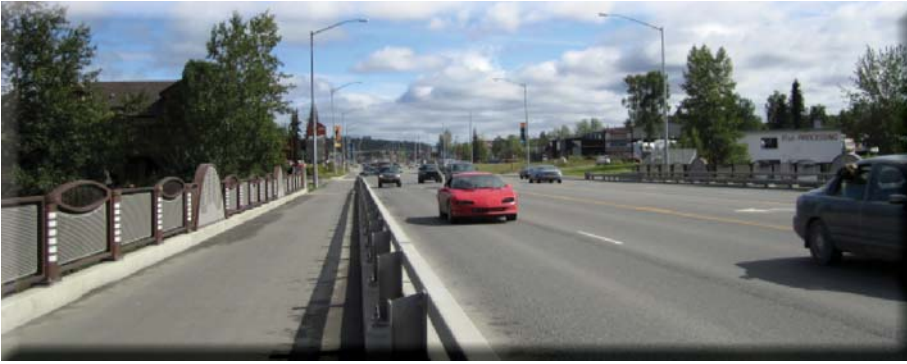
Sterling Highway can be difficult for pedestrians to cross
