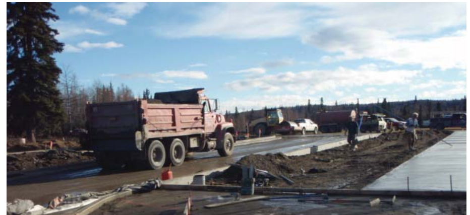
Crews work on upgrades to Soldotna Creek Park
