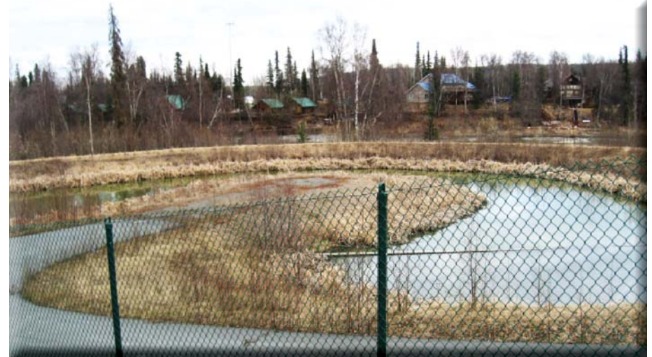
Storm water treatment system
