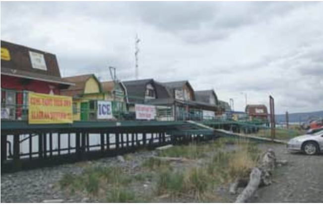
Commercial development on the Spit with specialty shops and restaurants connected by a boardwalk.
