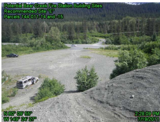
View looking east from the gravel pile
