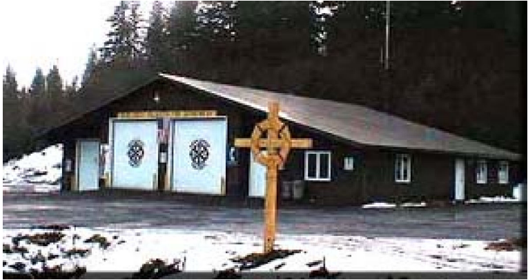
EXISTING FIRE STATION
