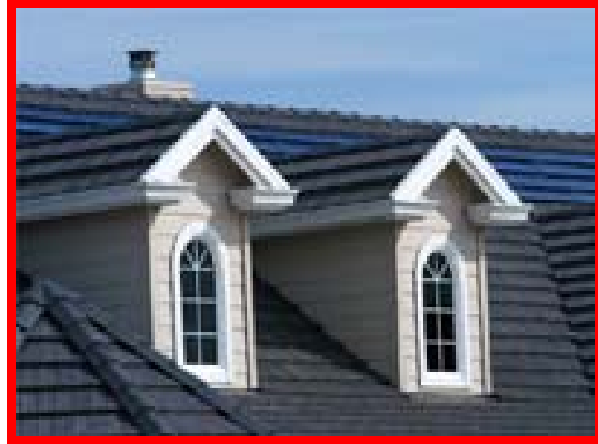
Solar Roofing Tile After Installation
