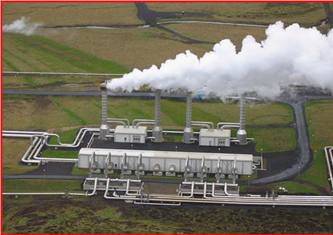
Geothermal Electricity Generation Plant in Iceland
