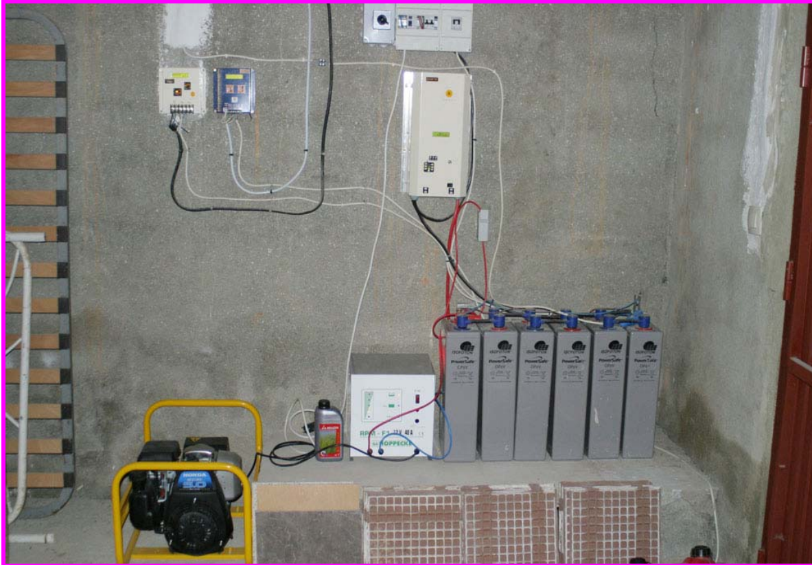
Typical Alternative Energy Battery Storage System
