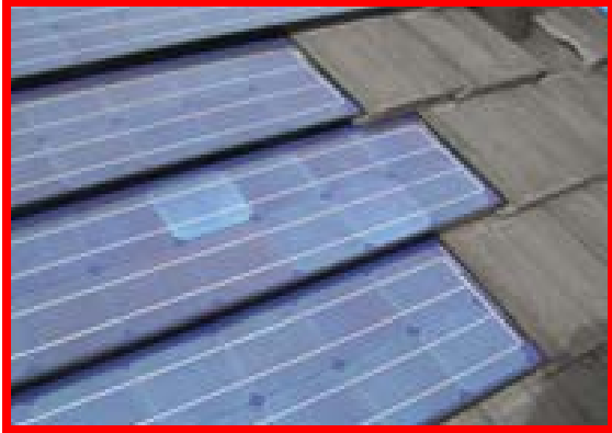
Solar Roofing Tile During Installation
