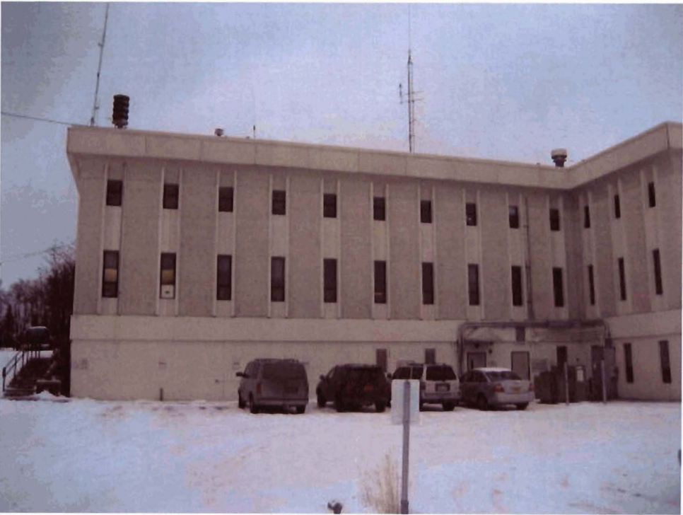
Photo 4: Proposed Location Next to Building for New Dry Coolers
